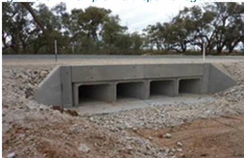
Figure 5-3 - Example multi-span bridge/culverts
